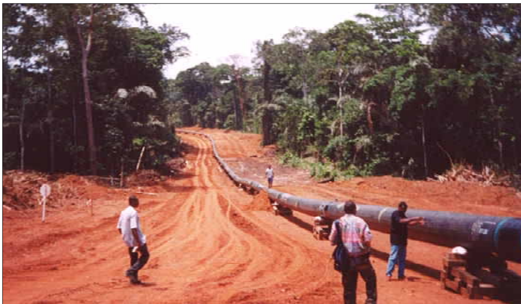
Pipeline during construction
