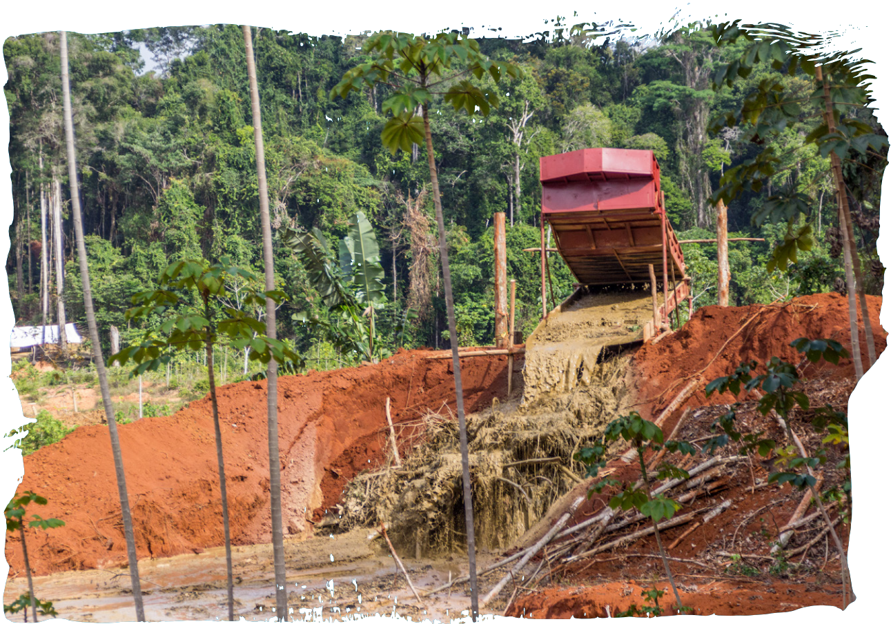
Sluicer pumping untreated water into an abandoned mine pit. Marudi Mine, South Rupununi, Guyana. Credit: Vicki Brown, FPP
