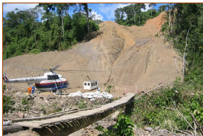
Rute jaringan pipa gas Camisea, lembah Urubamba © A Goldstein, 2003
